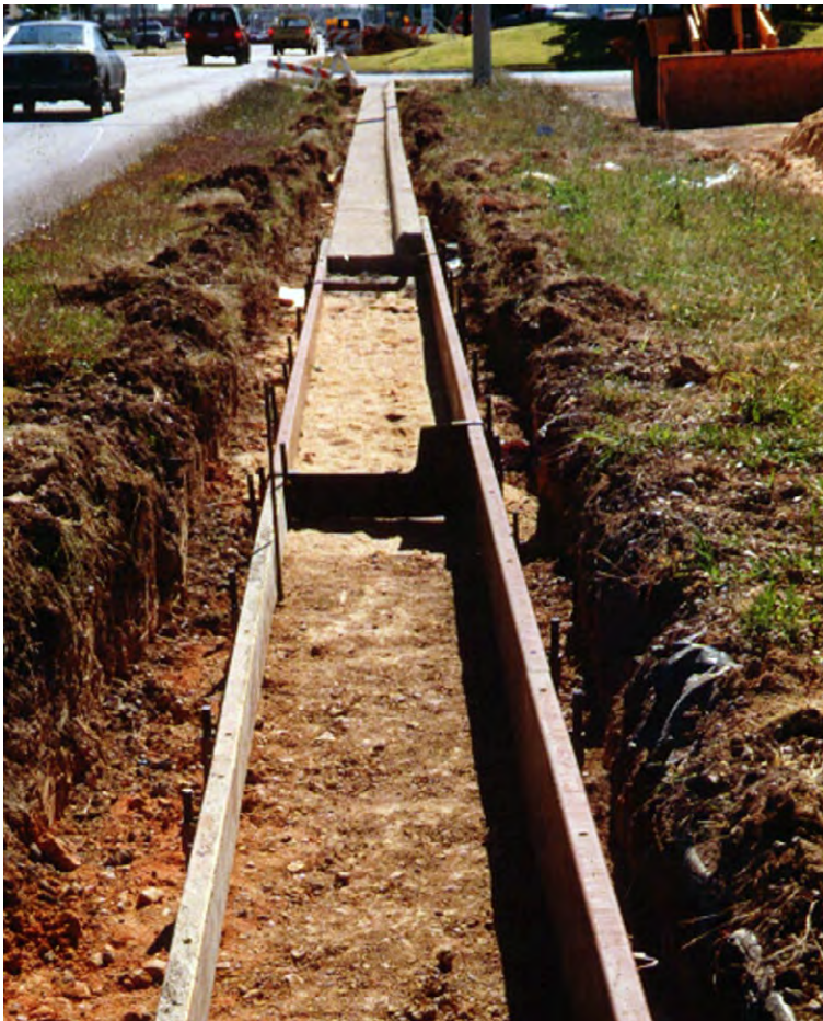
Hook the Division Plates over the front and back forms.
